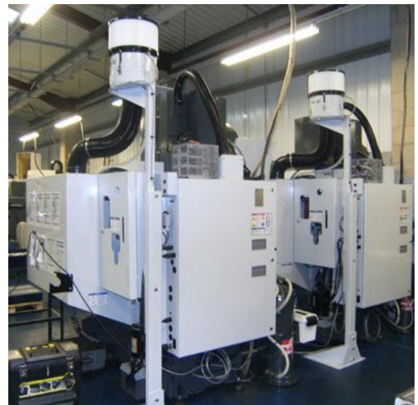
Filtermist Units Mounted on Floor Stands Next to Haas Minimills
